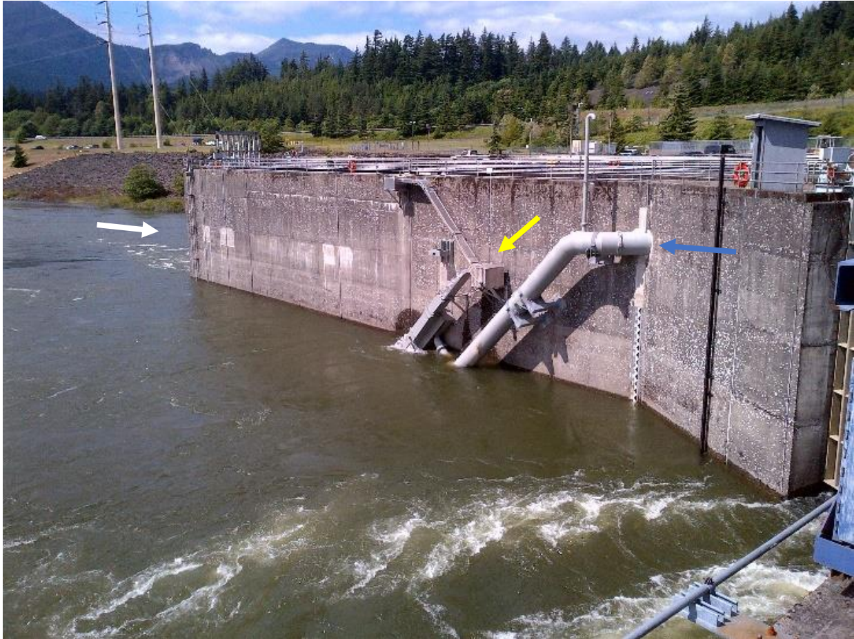
Figure 2. Lamprey Flume Structure (LFS) meets with rest box one (yellow arrow) and auxiliary attraction water grey pipe (blue arrow). Washington shore's north upstream fishway entrance at right and north downstream entrance (white arrow).
