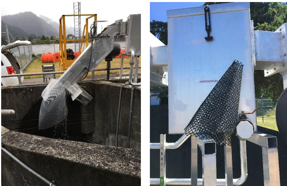
Figure 11. A cone of fish screen material was used to prevent lampreys from grazing the bridge wall or the opposing fishway wall (left image). Fyke that clogged with lampreys was removed from AWS upwelling box to allow fish to exit on 6/21/17 (right image).
